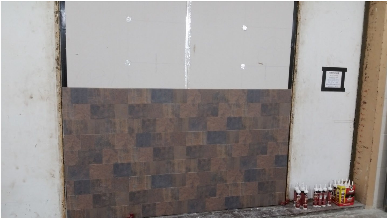
Figure 8 – Decorative wall panels partially installed on source room side
