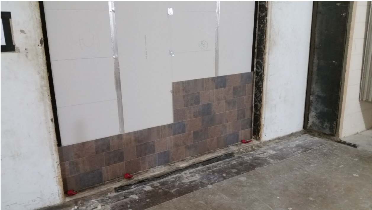
Figure 8 – Decorative wall panels partially installed on receive room side
