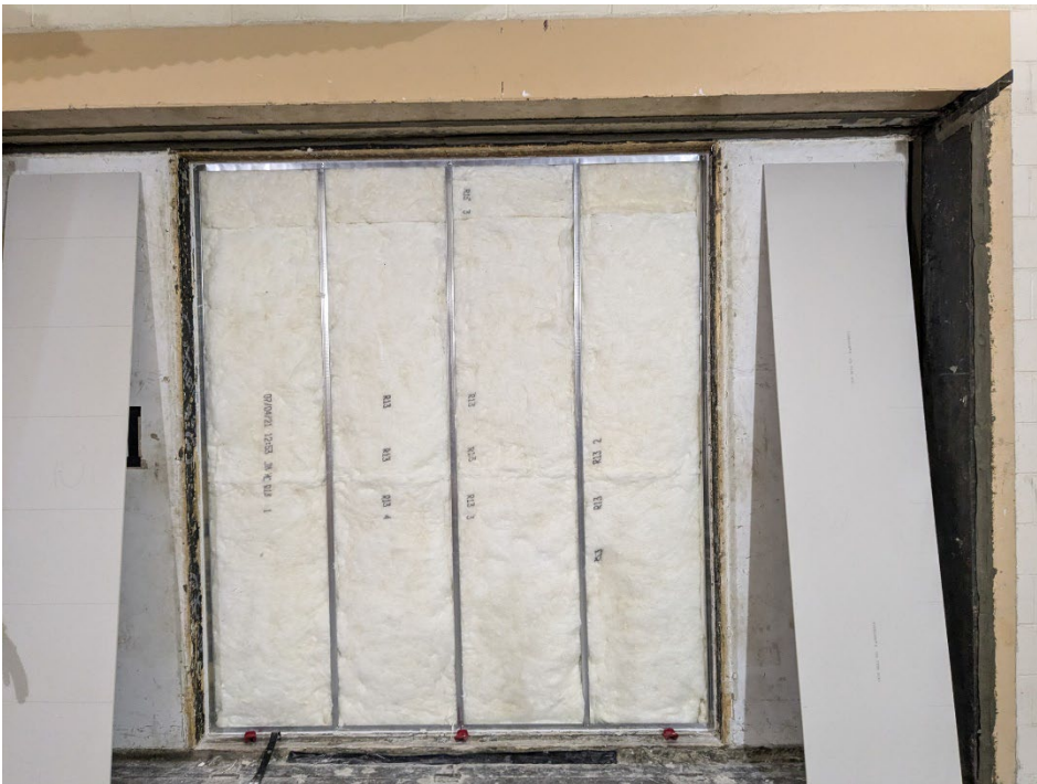
Figure 6 – Insulation installed in stud cavities
