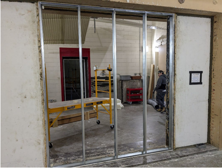
Figure 3 – Tracks and studs installed in test aperture
