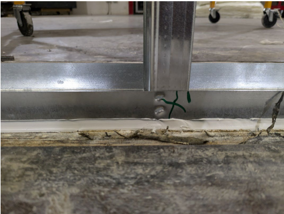
Figure 4 – Detail of stud double crimped to track
